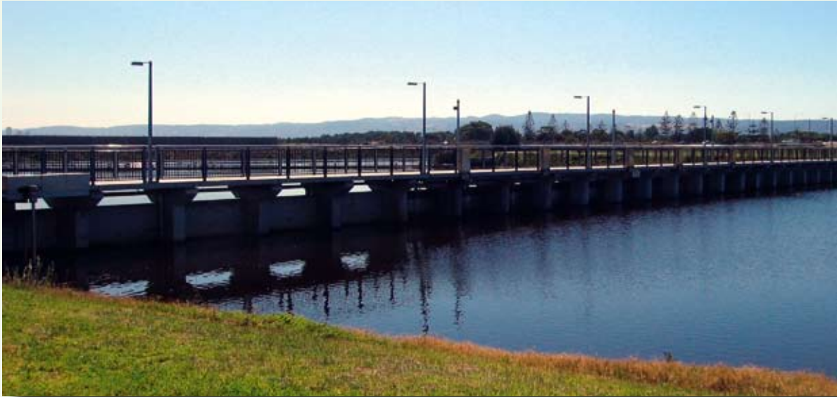
Diversion weir in the northern section of the Patawalonga Lake
